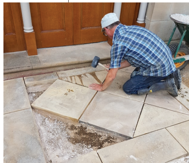
Flynn Stanton (above) excavating and Edrei Stanton (right) laying the stone threshold
